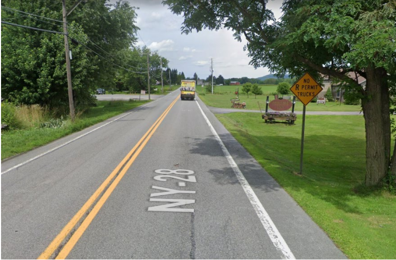
Figure 3 – Old Weight Restriction Postings on NY-28, South of Herkimer Creek.
