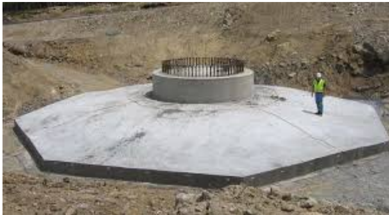
Figure 2: Shallow Foundation
